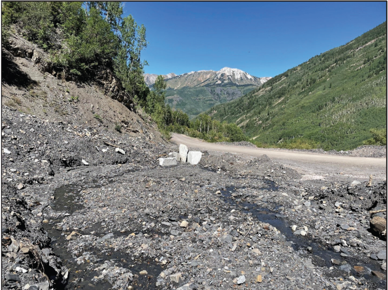
Figure 1. Braided slate deposition resulting from the July 21, 2021 mud slides at Mud Gulch along County Road 3c. White marble surrounds the current 42" culvert inlet. View to the north; photo captured August 24, 2021.
