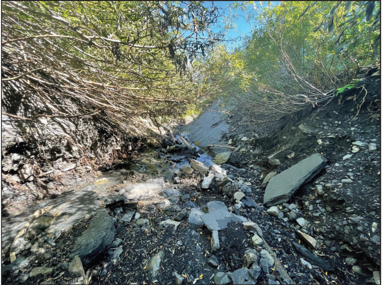
Figure 4. Existing channel slopes with bedrock Mancos Shale to the right and south with heavy vegetation throughout. View to the east; photo captured August 24, 2021.
