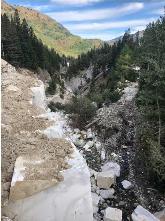
Photo 3. View north of the western alignment of Yule Creek (Photo: 8/30/18, pre-impact).
