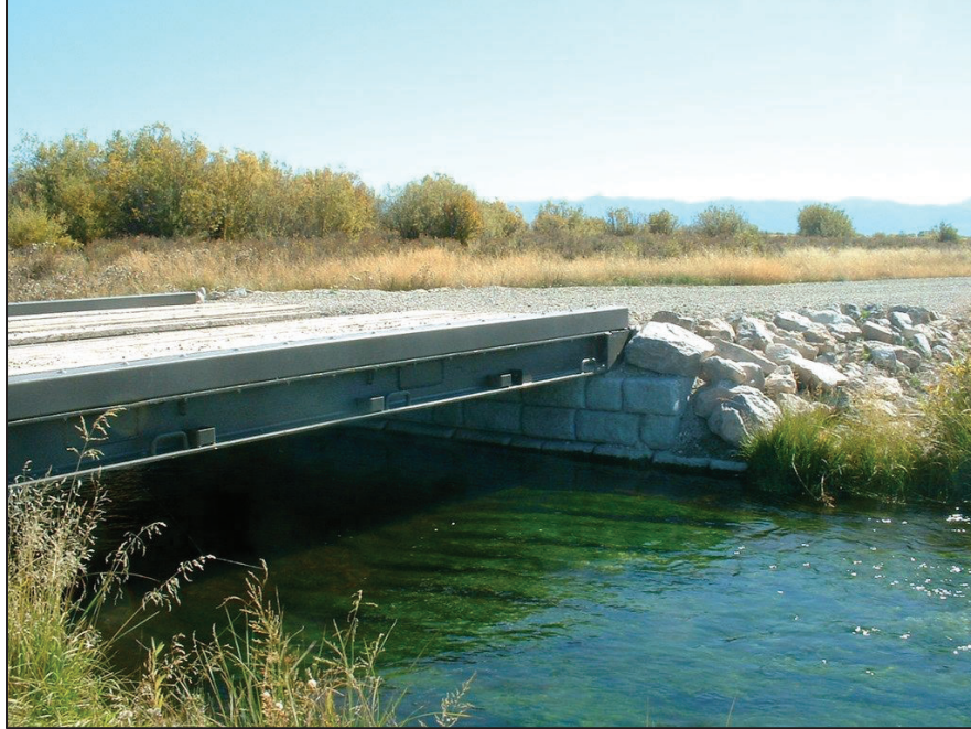
Figure 2. Example of a flatbed railcar bridge in use in Idaho courtesy of Redi-Rock. Note that the bridge is anchored in concrete while CSQ's crossing will use marble blocks.
